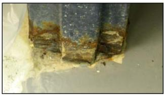
All doors and frames in this facility should be solid core, fiberglass systems that are gasketed and swept. It is very difficult to find any door system anywhere that has a combination of high STC (about 35 or better is ideal for a door) and long term tolerance of moisture. Additionally many shelters want to have some doors with glass in them. Chem-Pruf (www.chem-pruf.com) and Simon Door (www.frplite.com) are two options, but there are many fiberglass door manufacturers.
